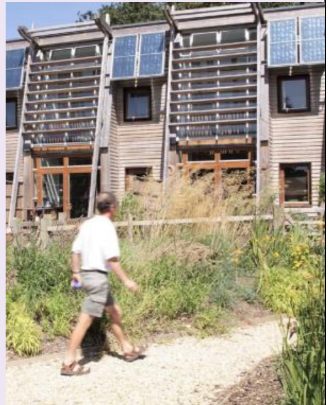
Figure 5: Example of window shades (National Design Guidance, CLG)
